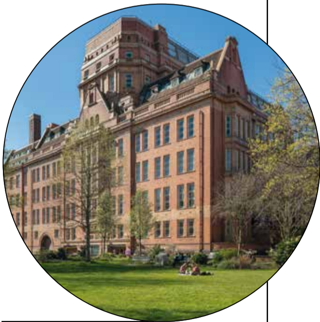
The Sackville Street Building
